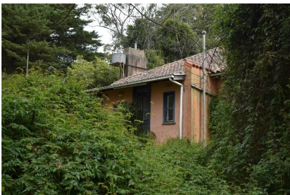
Figure 21. View of eastern section of the house from the northeast.
