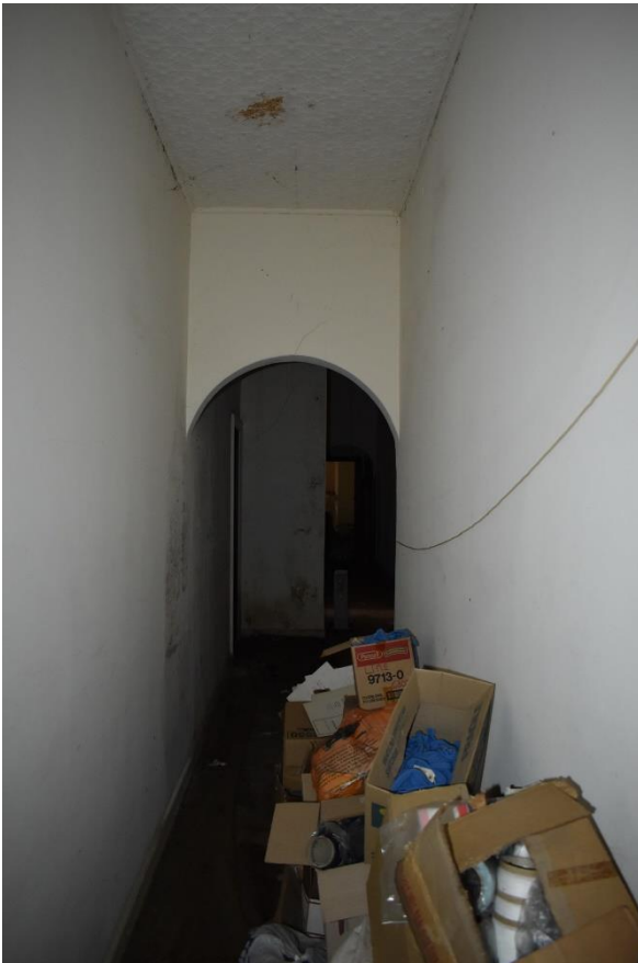
Figure 33. View of the pressed metal ceiling in the hallway.
