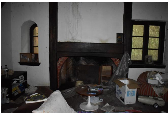
Figure 39. View of the fireplace and adjacent windows.
