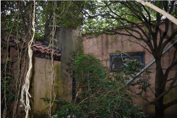
Figure 27. View of the wide, rectangular chimney from the courtyard.
