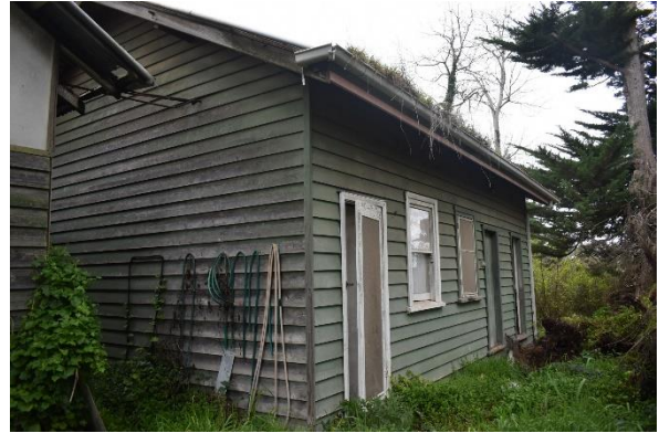
Figure 47. View of original Laundry.
