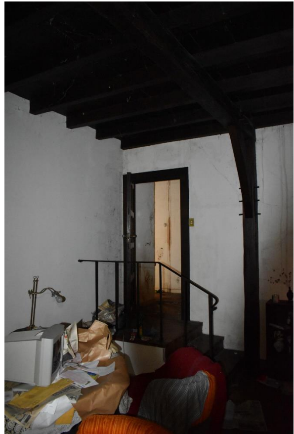
Figure 34. Interior view of the entryway to the Dining Room.
