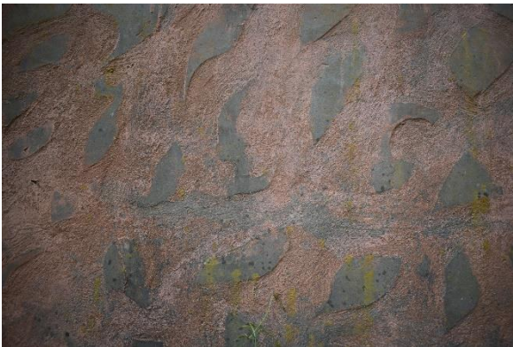
Figure 25. Detail view of the cement render.
