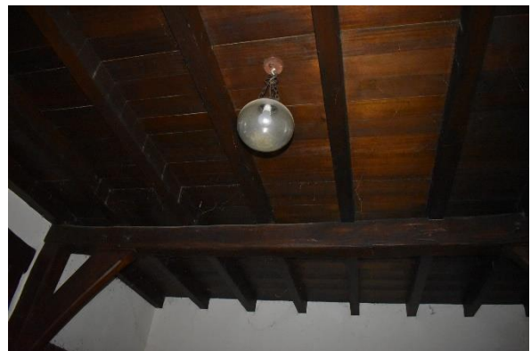
Figure 38. Detail view of the ceiling.
