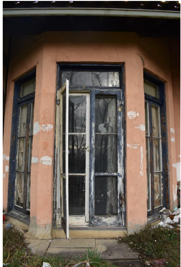
Figure 20. Detail view of the projecting bay to the northern elevation.
