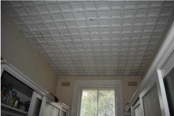
Figure 31. View of the pressed metal ceiling in the servery.
