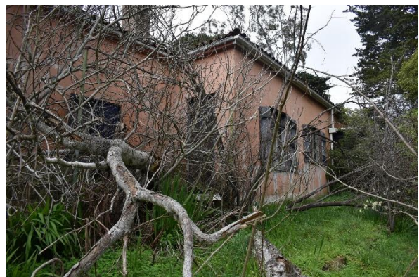
Figure 22. View of the eastern section of the house from the southeast.
