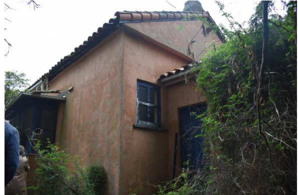
Figure 16. View of the western section of the house from the southwest.
