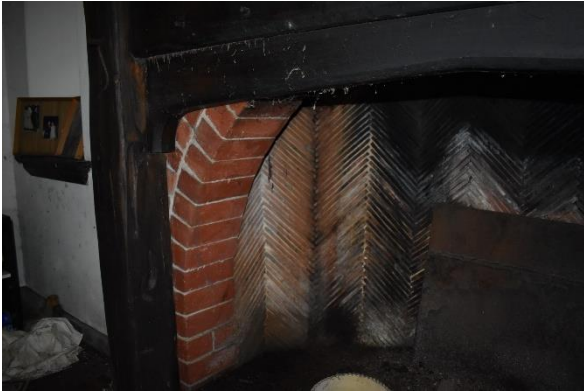
Figure 41. Detail view of the fireplace.
