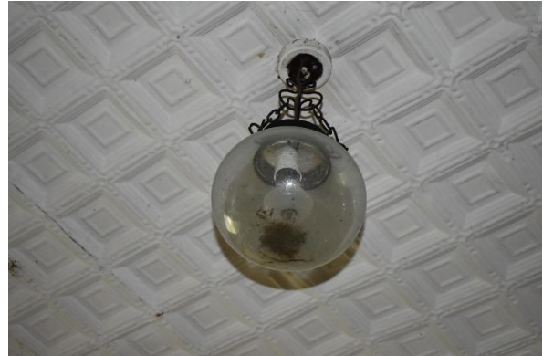
Figure 32. Detail view of the pressed metal ceiling and potentially an original light fixture.
