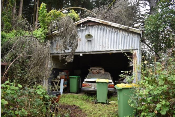
Figure 46. View of original double Garage.
