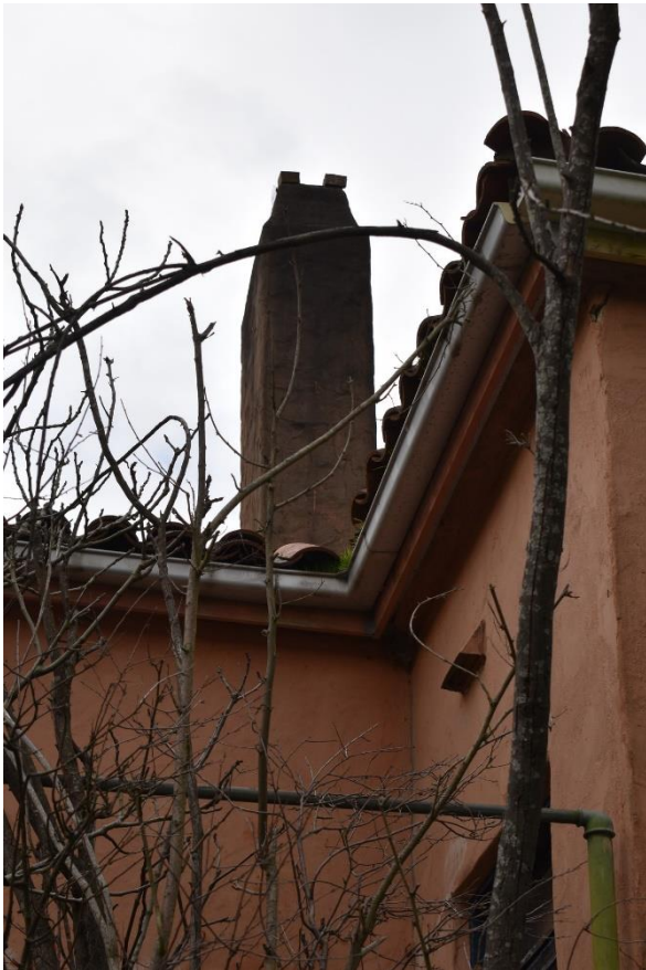
Figure 19. Detail view of a chimney.
