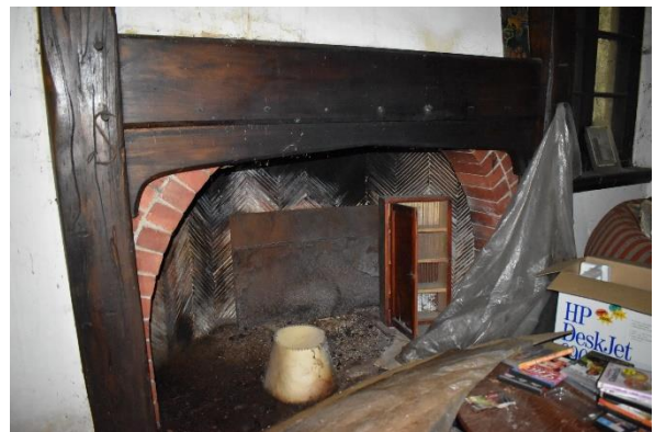
Figure 40. Detail view of the fireplace.
