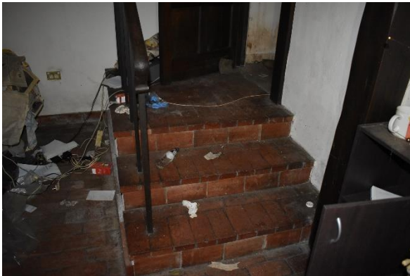
Figure 35. Detail view of the stairs in the Dining Room.
